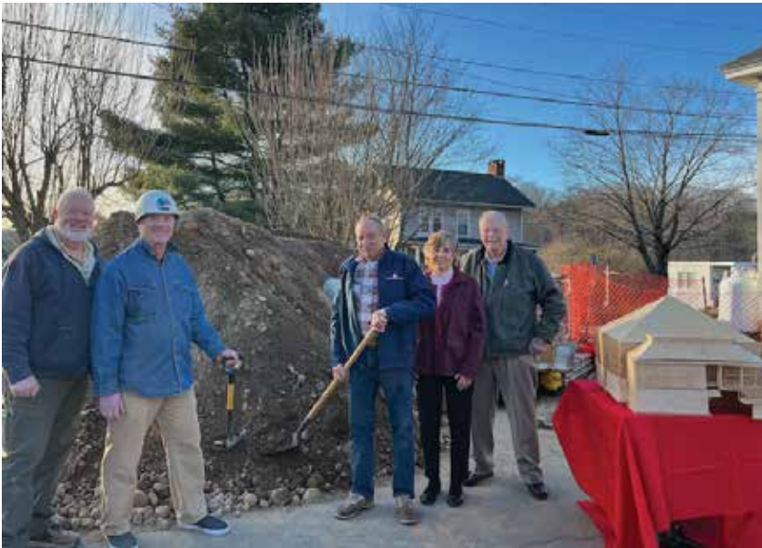
PHOTO CAPTION: (from l-r) Essex Veterans Memorial Hall members Paul Knudsen and John Lee, with The Essex Foundation board members Strickland Hyde and Judy Bombaci, and EVMH President Art Davies break ground on the Hall's expansion and renovation project funded by a community matching gift effort and in-kind donations. A model of the finished expansion work is displayed to the right.
