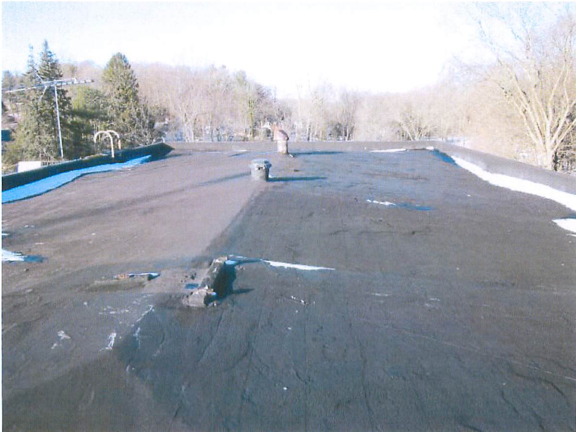
Main roof looking north along the East wing.
