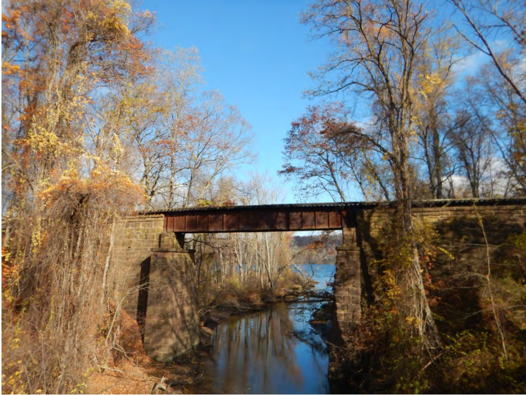
Mill River Bridge (MP 14.74)
