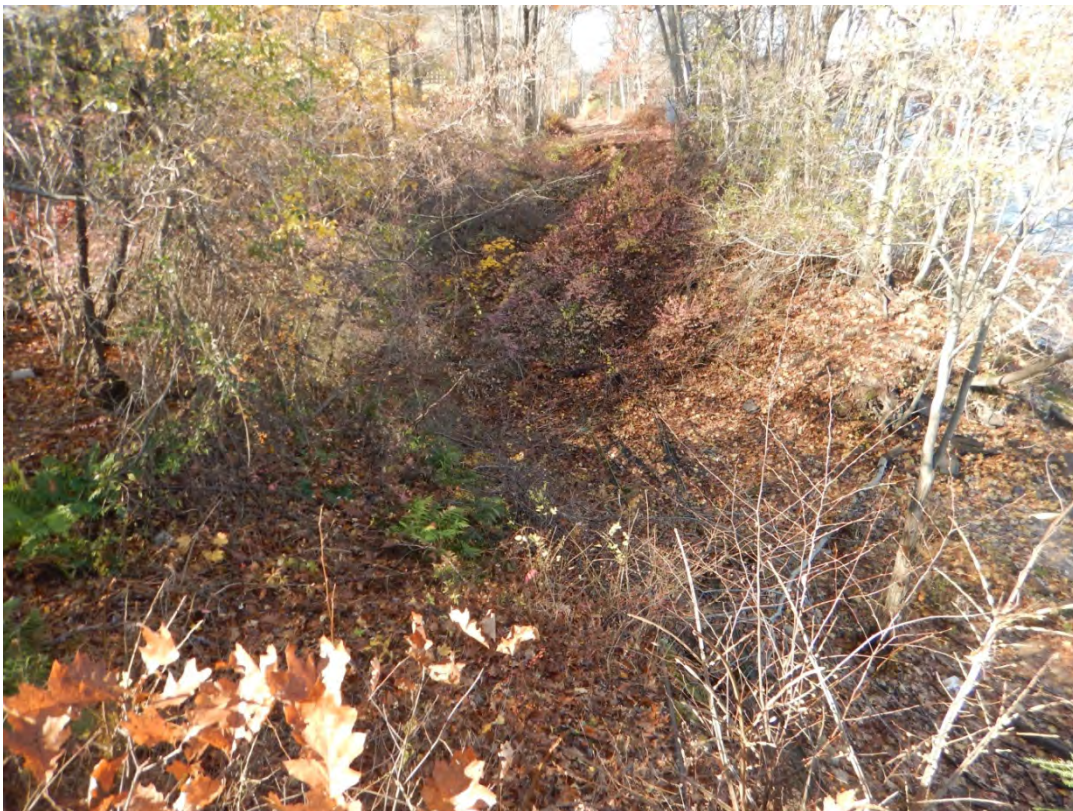
Washout along the line (MP 17.67)
