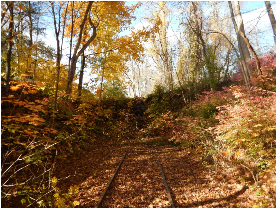
Driveway embankment constructed across line (MP 14.4)
