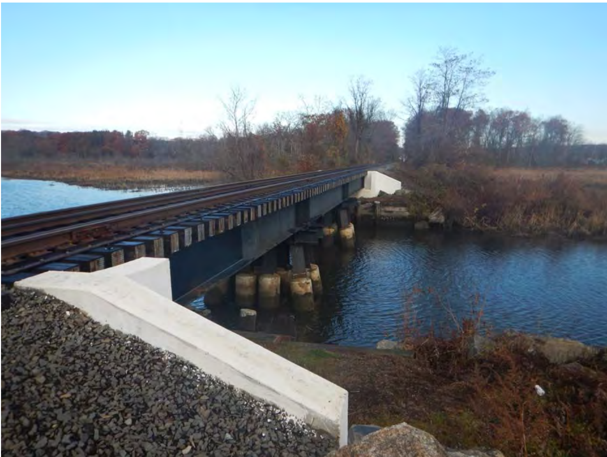
Bridge over the Deep River (MP 8.15)
