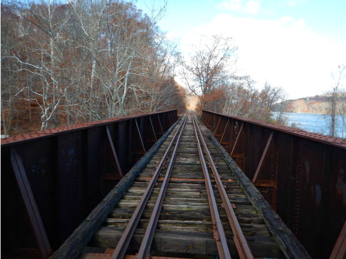
Higganum Cove Bridge (MP 18.48)
