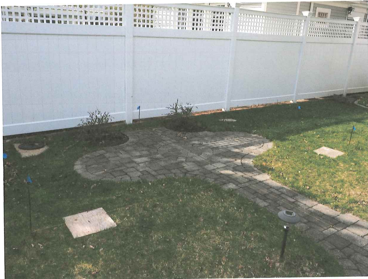
PERGOLA FOUNDATION HOLES (COVERWED)
