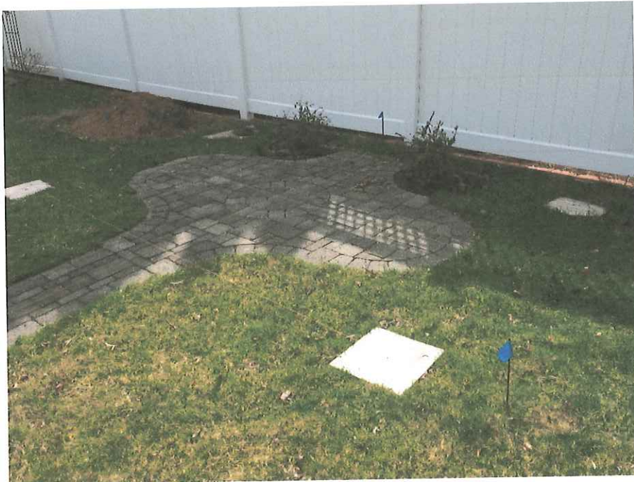
PERGOLA FOUNIDATION HOLES (COVERWED)
