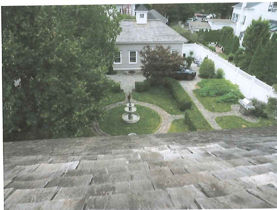
PARTIAL BACK YARD FROM ROOF HATCH
