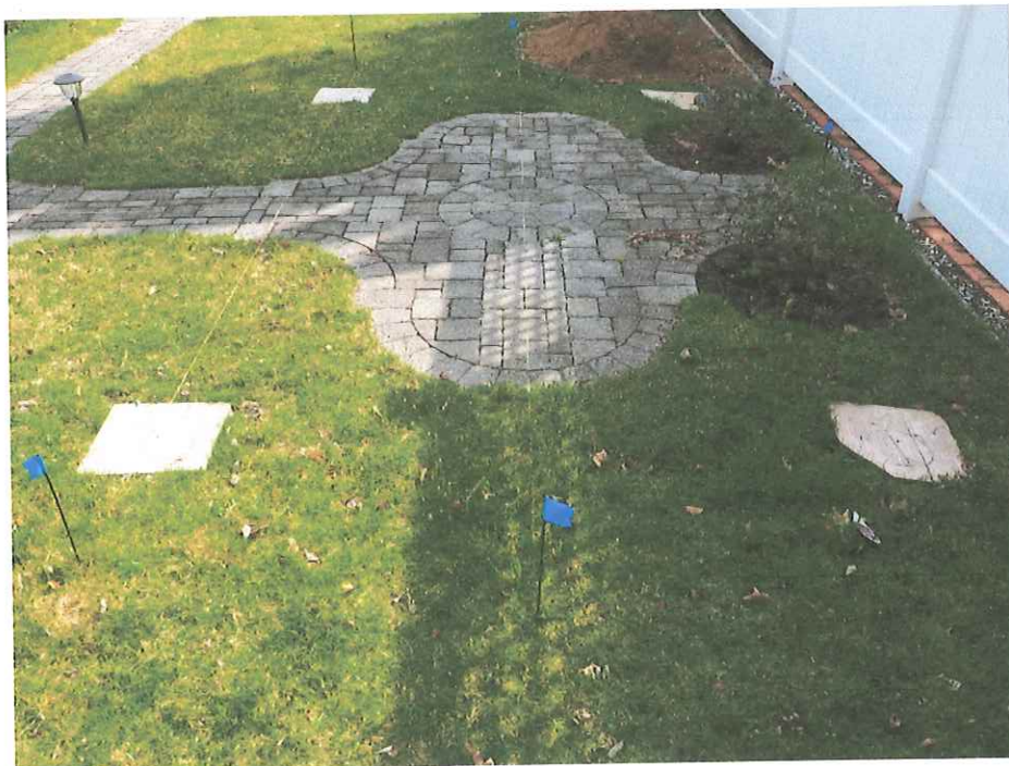
PERGOLA FOUNIDATION HOLES (COVERWED)
