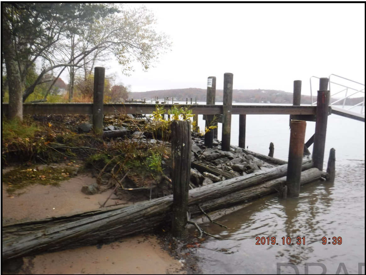
View of shoreline and structures looking upriver.
