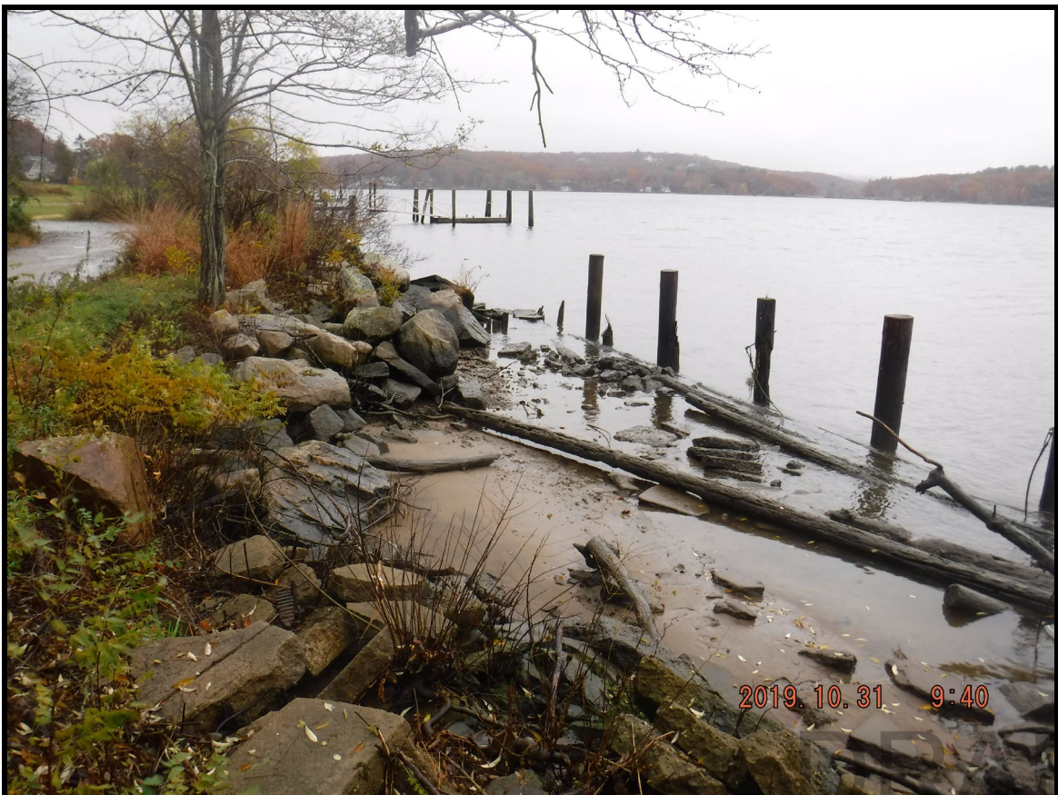
View shoreline and timber bulkhead remains looking upriver.
