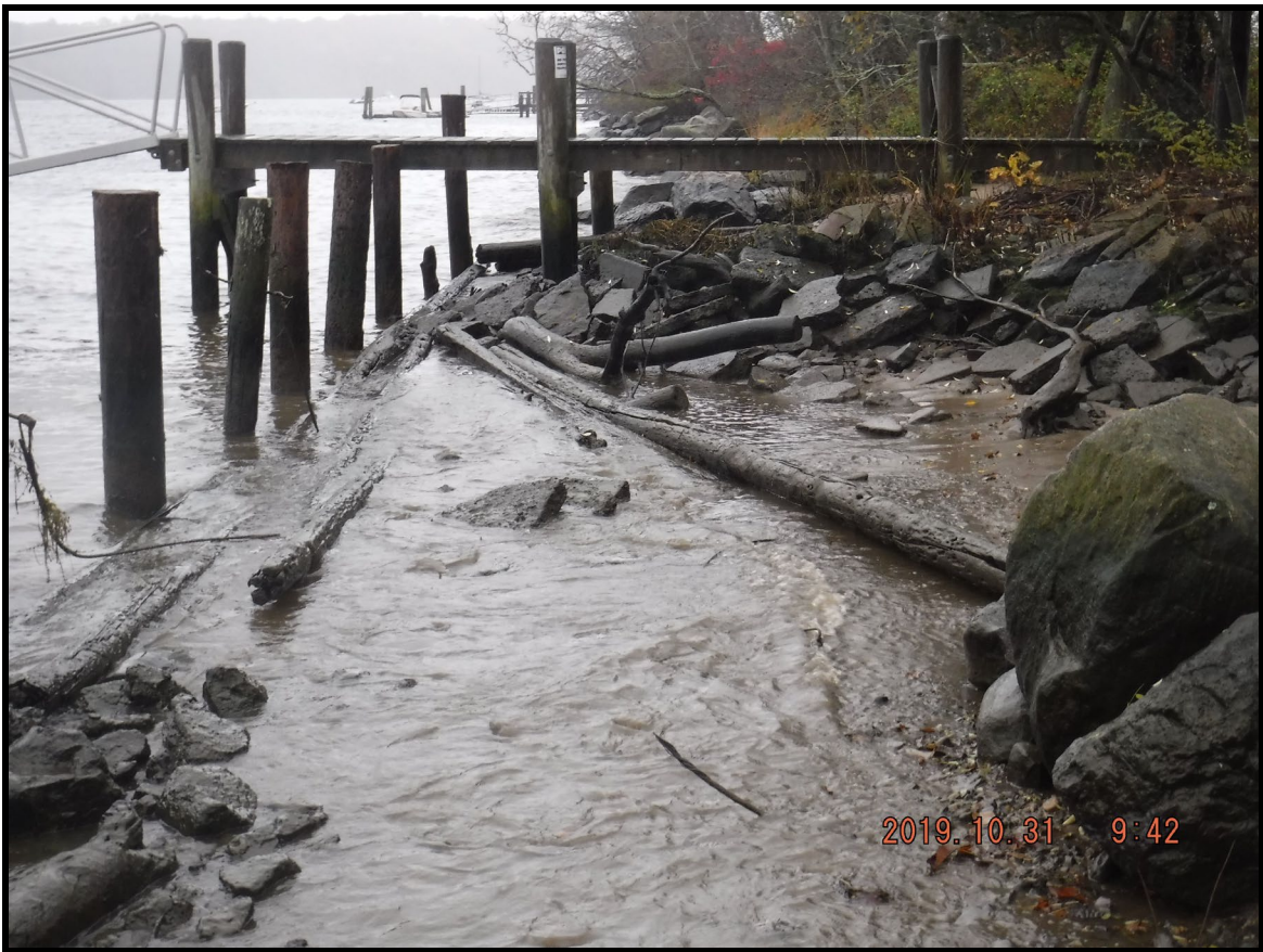
View of timber bulkhead remains and pier looking downriver.
