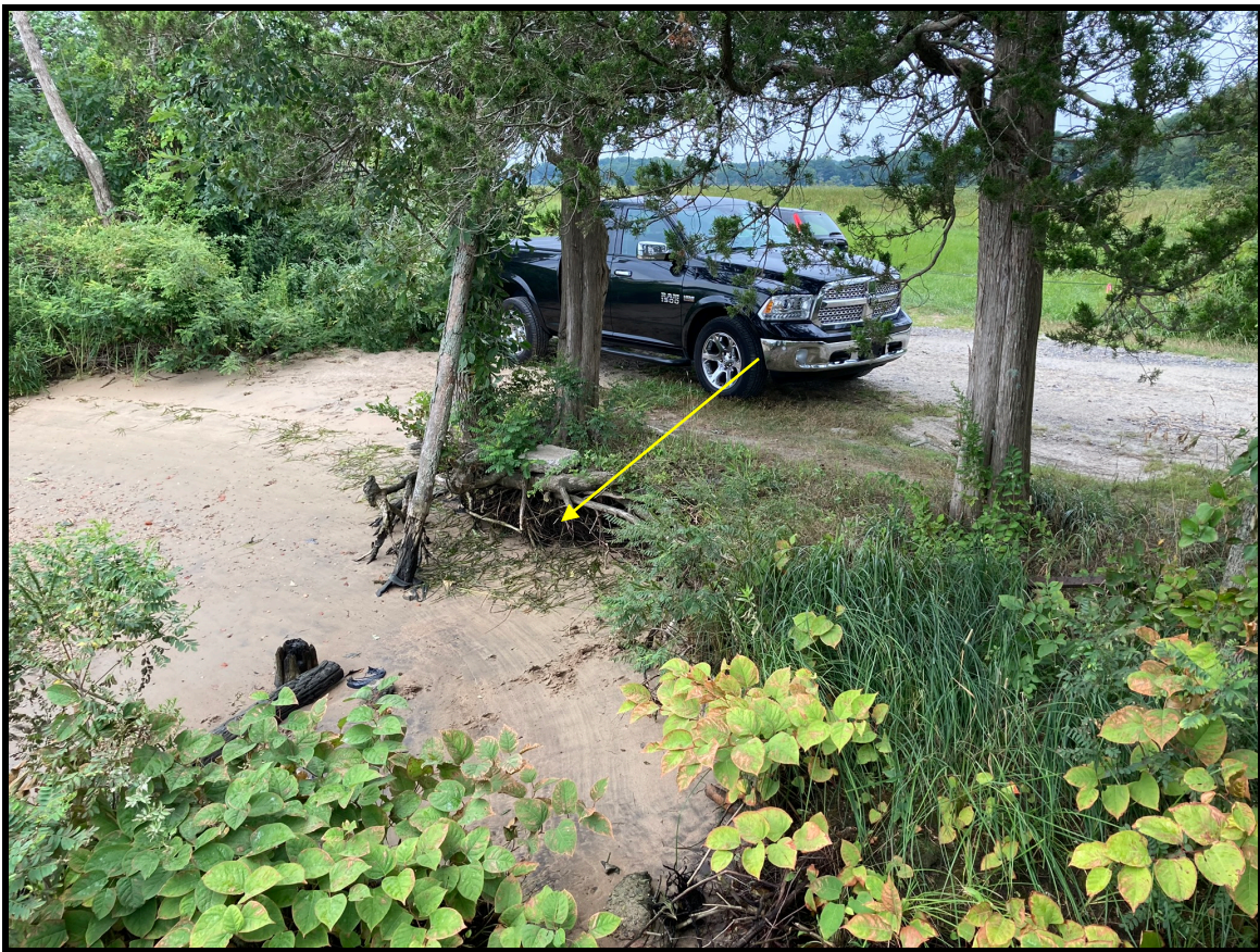
View of eroding shoreline near boat launch area and access drive.
