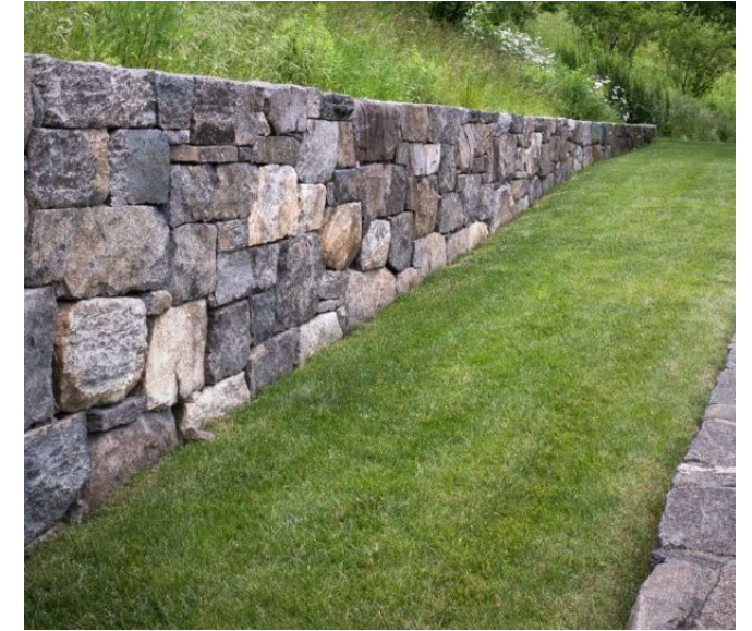
CT STONE, DRY LAID
